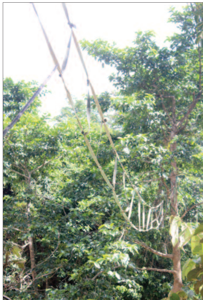
Close-up of the bridge over Sungei Pin.
